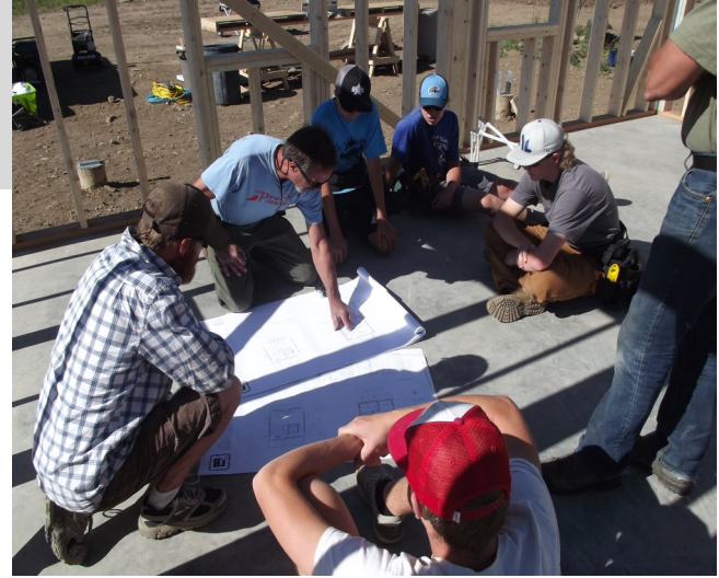
Crested Butte students and community members working on the Community School Town Rental Build project, building a rental unit for Town of Crested Butte employees.
