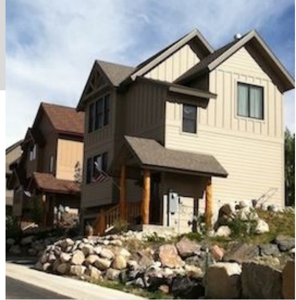
Hideaway Place Apartments
