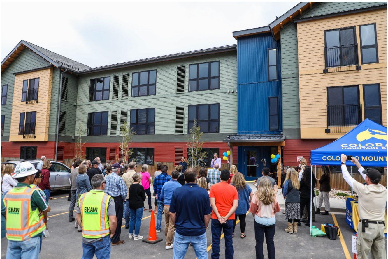
People gather Tuesday for the official dedication of the new Colorado Mountain College Vail Valley apartments in Edwards. Two buildings have been built, one funded by the school and the other by Eagle County. Chris Dillmann/Vail Daily
